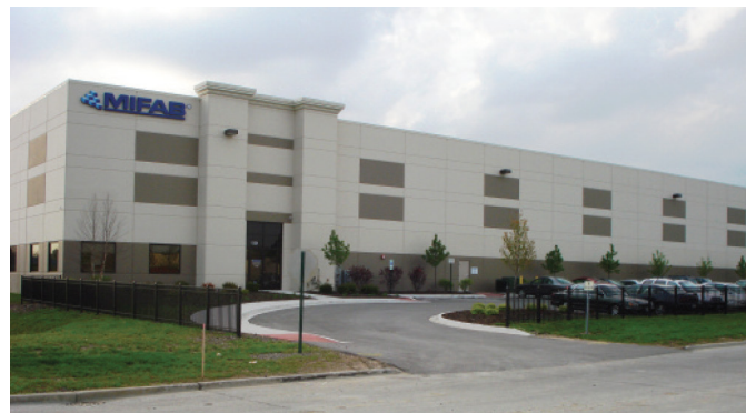
MIFAB's factory in Chicago, Illinois
